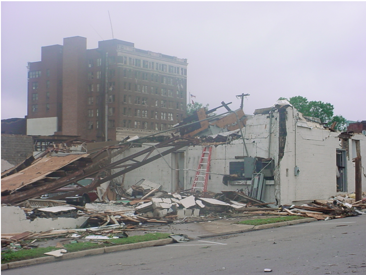
Figure 1: May 4, 2003 tornado damage in Jackson, TN.
